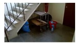
In the old Oceanography building, items were being stored under one of the stairwells. Although most was not combustible, this area should not be seen as a storage place. Escape stairwells should be seen as sterile areas and be kept clear.
