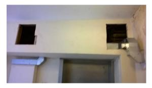
During the assessment, new electrical switchgear had been installed on the north stairwell and some holes were noted. FRCS have confirmed that this equipment will be boxed in with 1 hour fire protection material and locked off.
