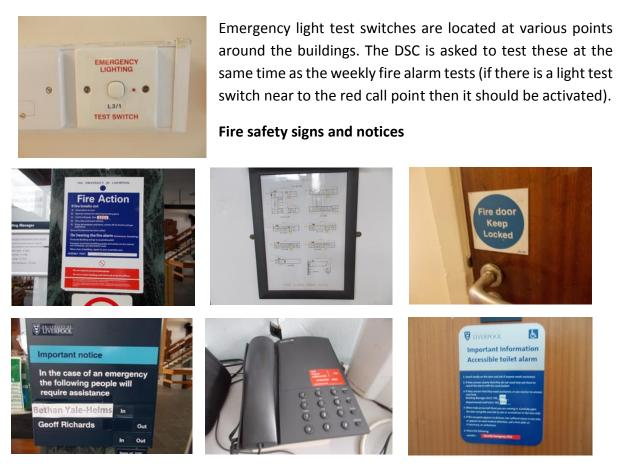
Generally, the standards of signage were good. The panel had a clear mimic diagram to indicate the relevant zones, directional signage was fitted, fire action notices were located near call points and clear mandatory signage was in place for fire doors, etc. Signage for final exit door operation was also fitted and clear. There was evidence of emergency number stickers on telephones and accessible toilets had the standard emergency contact number signs displayed.
