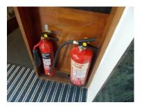
There were an adequate number of fire extinguishers in the two blocks. Normally found in pairs but occasionally as a single unit, they were foam and CO2. It was not considered necessary to provide further extinguishers in the area.
