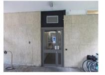
The vast majority of areas were fitted with adequate emergency lighting. This was both on internal stairwells and corridors and on external doors. The only areas were additional lighting was considered necessary was above the doors below (i.e. two single doors out of ground floor lecture theatre (South side) which appeared only to have standard light fittings in the vicinity):
