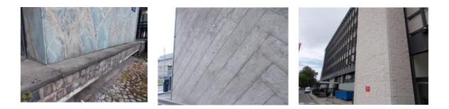
The main tower is constructed from a number of materials but is essentially a brick/metal frame building with concrete, stone and wood panelling fitted across various sections. The building has a significant amount of glazing on the two main sides of the tower. Both buildings have flat roof areas.
