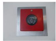
The Fire Service should note that the lift in the North stairwell is fitted with a fireman's control switch.
