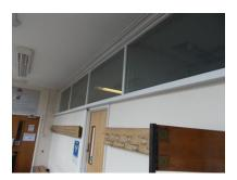
Second floor – most of the offices in the tower have escape in two directions. One end of the building has escape in one direction. As travel distances are close to 18m the space outside the main lecture theatre has been fitted with fire resistant glazing suggested that this route is now protected (a previous assessment in 2003 suggested this as an option for these spaces).
